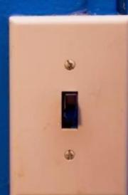
A photograph of a single-pole light switch mounted on a blue wall. The switch is a standard toggle type with a black handle.
