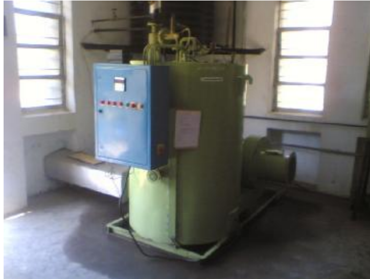
'ECOTHERM 600' : Diesel fired, fully automatic, water tube steam generator
